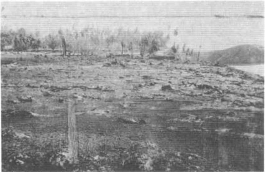
Angahâ village destroyed, 1946. Tongan photos bureau
